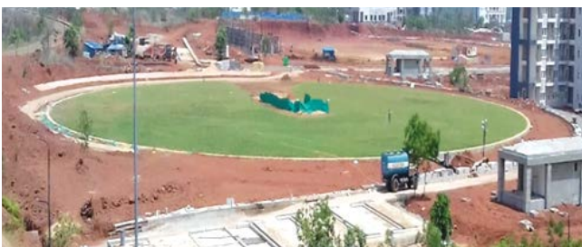
Cricket Ground: Finishing work is in progress.
