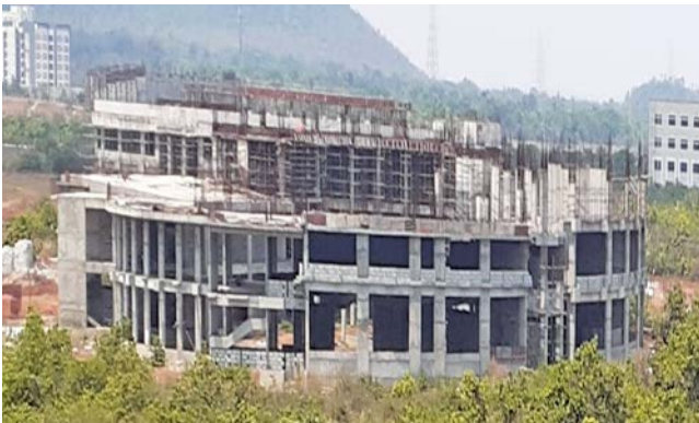
LTC-1: Structural work completed.
