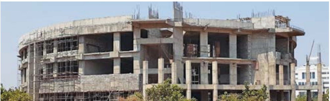
LTC 3: The structural work completed.
