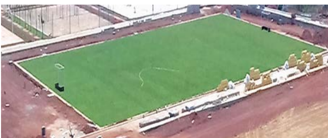
Hockey Ground: Finishing work is in progress.
