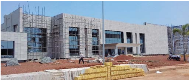
Student Activity Centre: Finishing work is in progress
