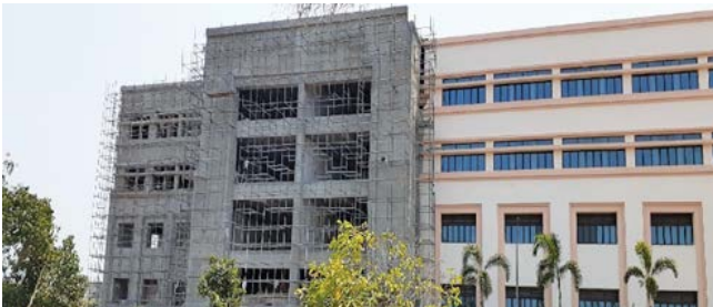
SBS Extension: The structural work completed & finishing work is in progress
