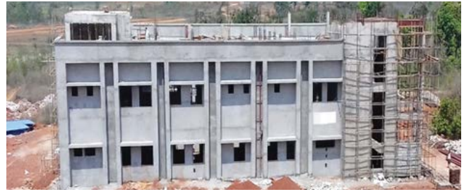
Dispensary: Finishing work is in progress.
