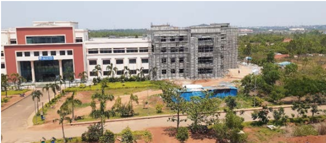
SIF Extension: The structural work completed & finishing work is in progress.
