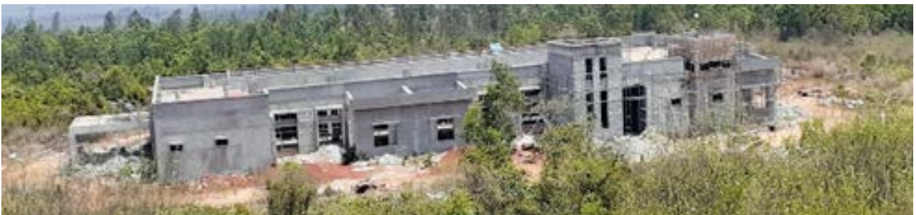
Central Workshop: The structural work completed & finishing work is in progress
