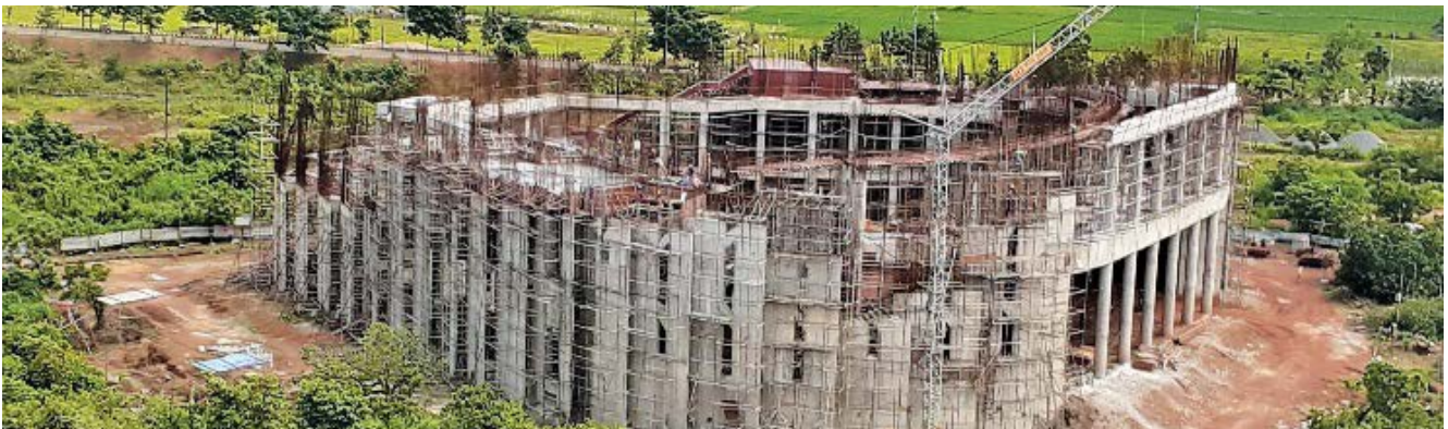
Auditorium: Structural Work of 1 st floor is in progress
