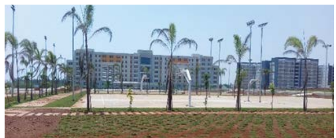
Basketball, Volleyball and Tennis Court : Finishing work is in progress.
