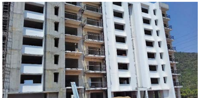
Type-D1 & D2 Quarters: Finishing work is in Progress
