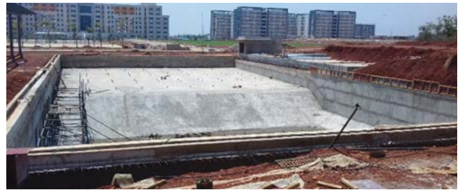
Swimming Pool: Finishing work is in progress
