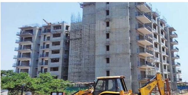
Type- C3 Quarters: Finishing work is in progress.
