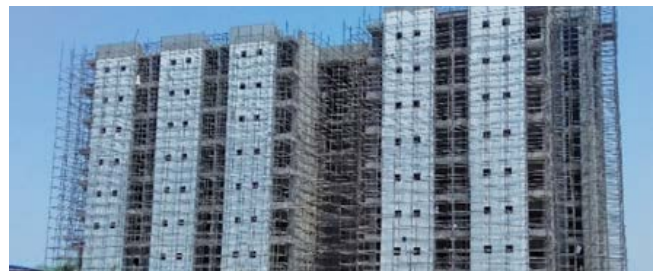
Efficiency Hostel: Finishing work is in progress
