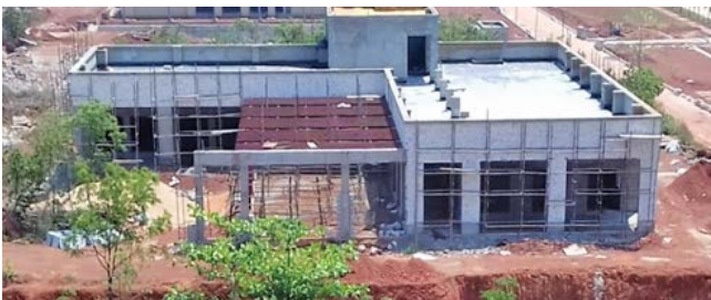
Commercial complex (Res): Finishing work is in progress.
