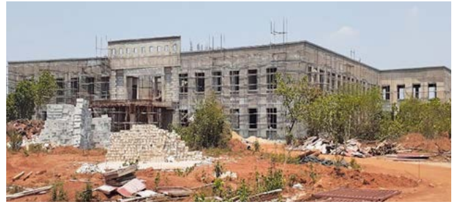
SEOCs: The structural work completed & finishing work is in progress.
