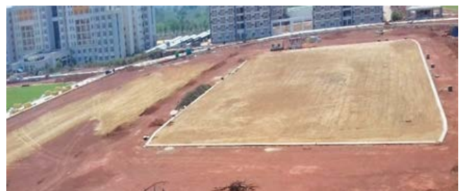
Football Ground with the athletic track: Work is in Progress.
