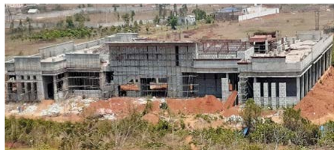
CRIF: Work completed & finishing work is in progress
