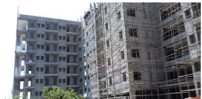
Boys' Hostel-3: B wing finishing work is in Progress
