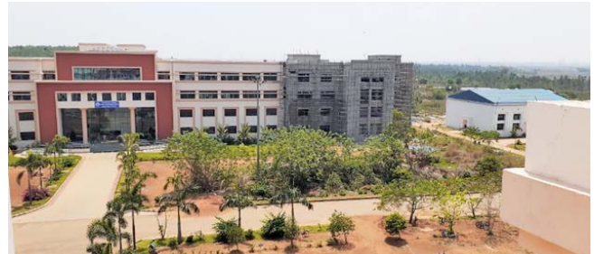
SMS Extension: The structural work completed & finishing work is in progress.
