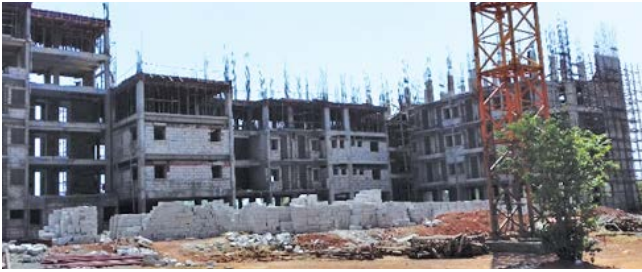
Boys' Hostel-3: A wing 3 rd floor roof slab completed.
