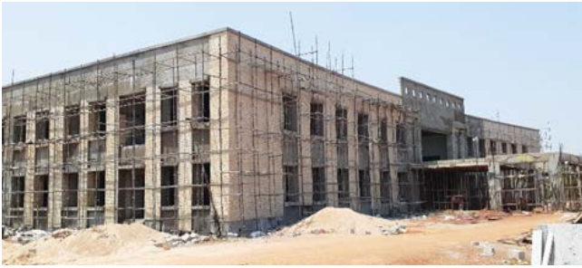
SMMME: The structural work completed & finishing work is in progress
