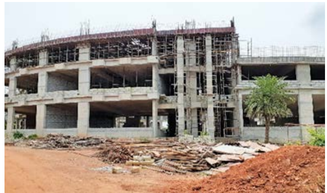
LTC-2: 2 nd floor roof slab work is in progress
